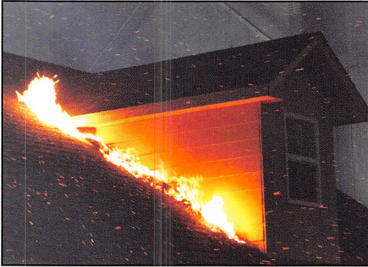
Debris can build up in corners, providing fuel for embers. Photo by Institute for Business and Home Safety Research Center.
