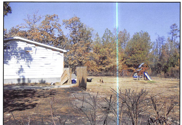
This home escaped the flames when firefighters knocked down the burning fence that would have led flames to the home. Notice the burn marks on the fence.
