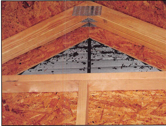
Screening helped capture these embers and prevent their entry into the attic. Photo by Institute for Business and Safety Research Center.
